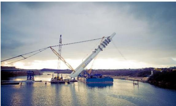
Figure 1. Bridge pylon during erection, February 2017.
